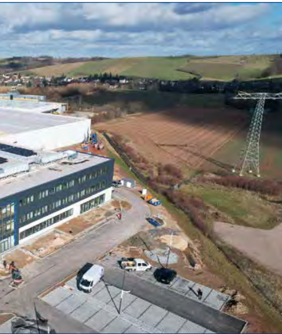
The new company complex of AKE Systemtechnik GmbH, in the industrial park Reinsdorf near Zwickau, in its final stage of development at the end of February 2022. The move from the old location to the new building will take place on schedule in the second quarter.
