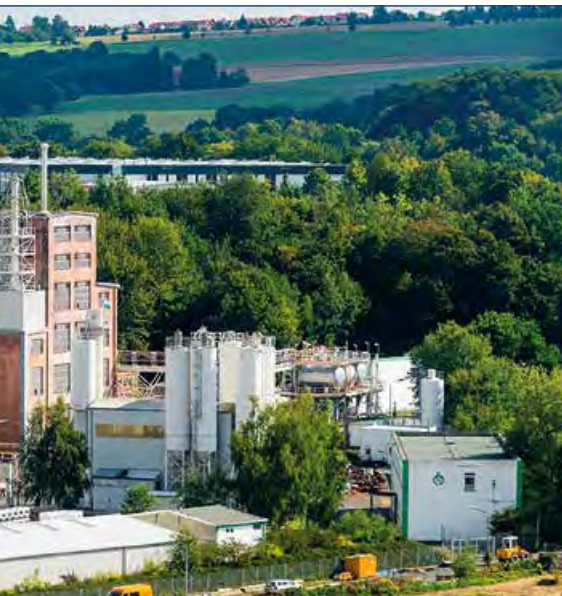
Great changes lie ahead at the Fluorchemie Dohna premises in the coming years. The company is planning to make extensive investments in order to boost its production of hydrofluoric acid, a key substance for the electrolyte in lithium-ion batteries.
